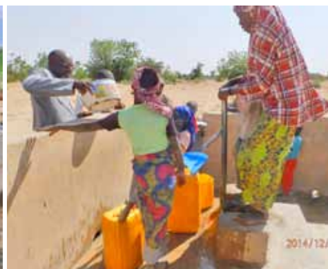
Renovated pump well in Garin-wali Village
