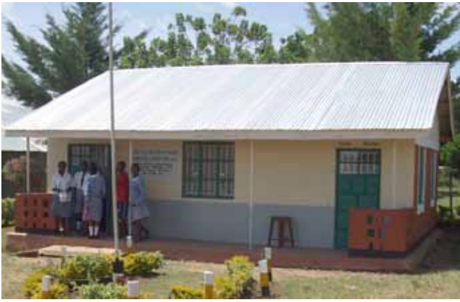
Newly built computer classroom
